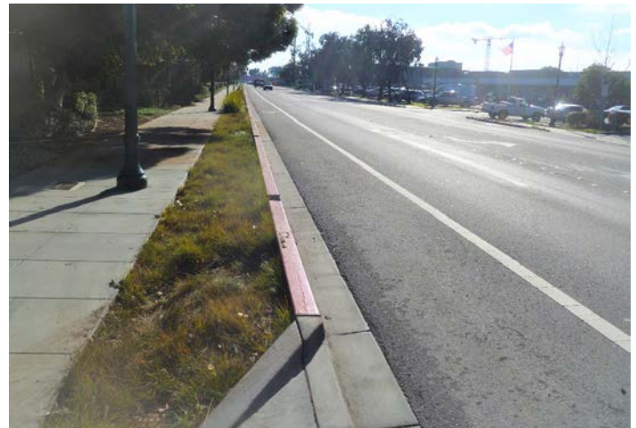
PHOTO SHOWS VIEW ON DELAWARE STREET FACING SOUTH TOWARDS THE POST OFFICE, HIGHLIGHTING THE BIOSWALES BESIDE THE WIDENED SIDEWALKS.
