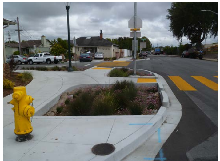
PHOTO SHOWING INTERSECTION WITH BIOSWALE BULB-OUTS
