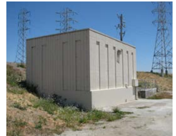
POPLAR AVENUE EXISTING STRUCTURE
