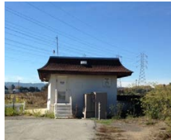
COYOTE POINT EXISTING STRUCTURE
