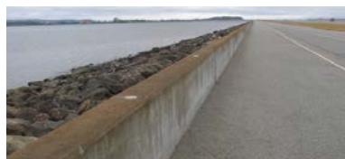
EXISTING CONCRETE WALL WITH RIPRAP PROTECTION AT R11-28R
