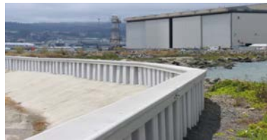
EXISTING DIKE AND VINYL SHEET PILE PROTECTION AT R7-19 ENDS
