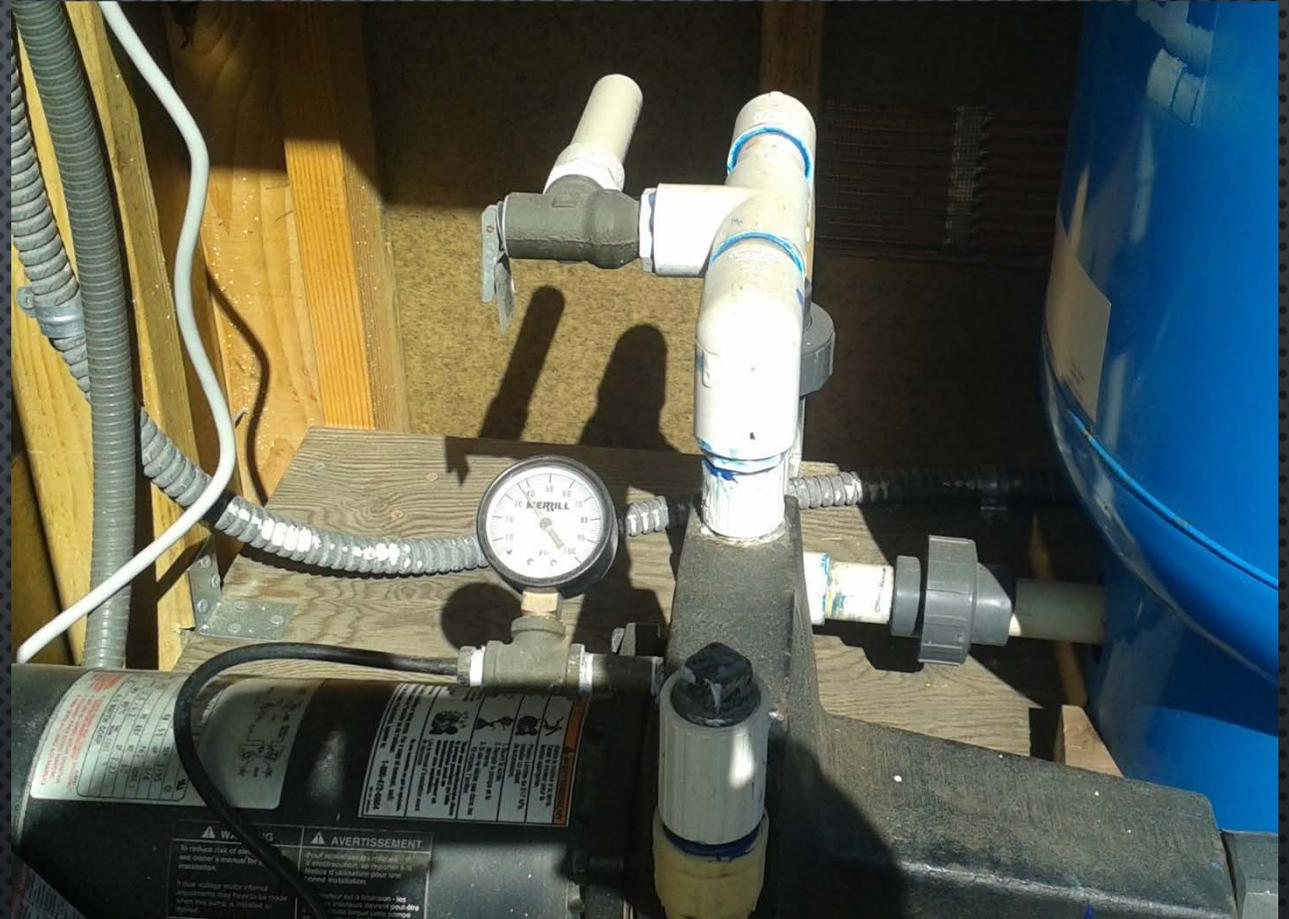
Simple pump system switches on at low pressure in storage container, off at higher pressure
