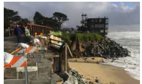
Erosion at Mirada Rd. Photo credit: Office of Sustainability.
