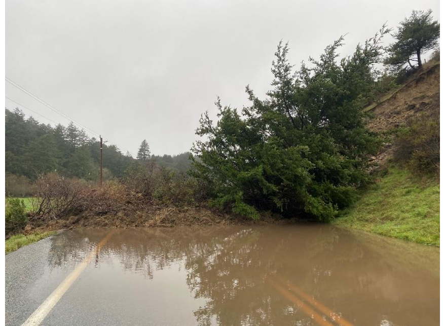
Cloverdale Road – Slide/Debris Removal
