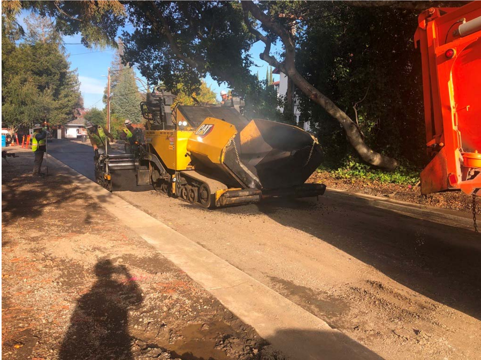
Paving first lift of AC after cement treatment of base
