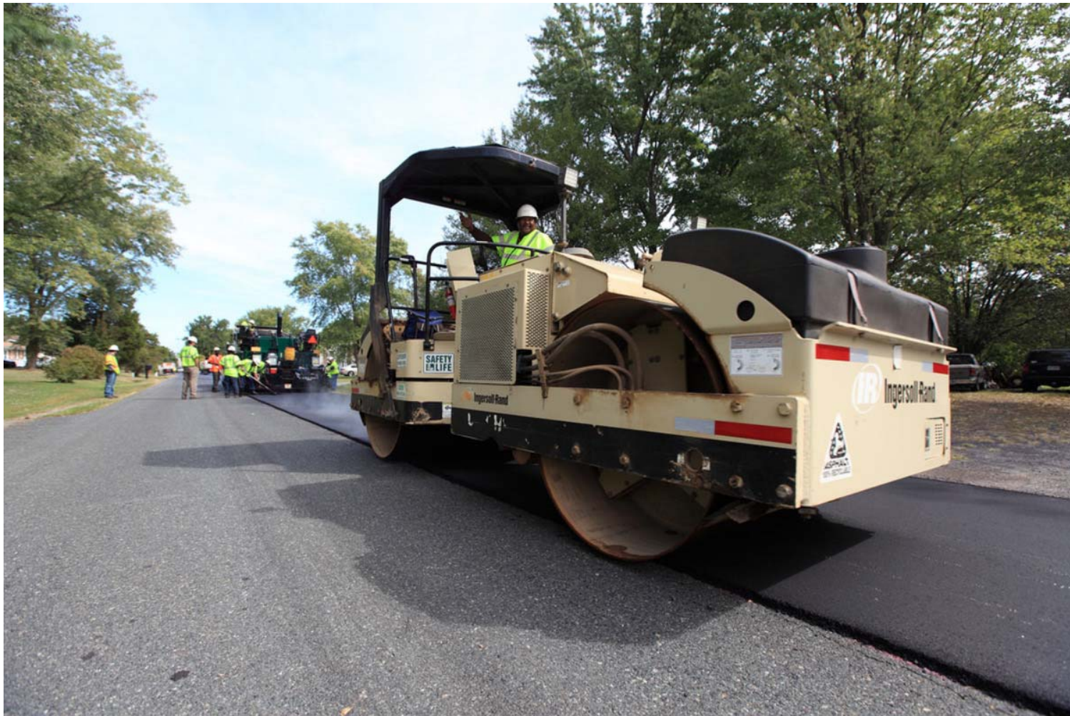
Drum Roller – Rolling AC after placement by paving machine
