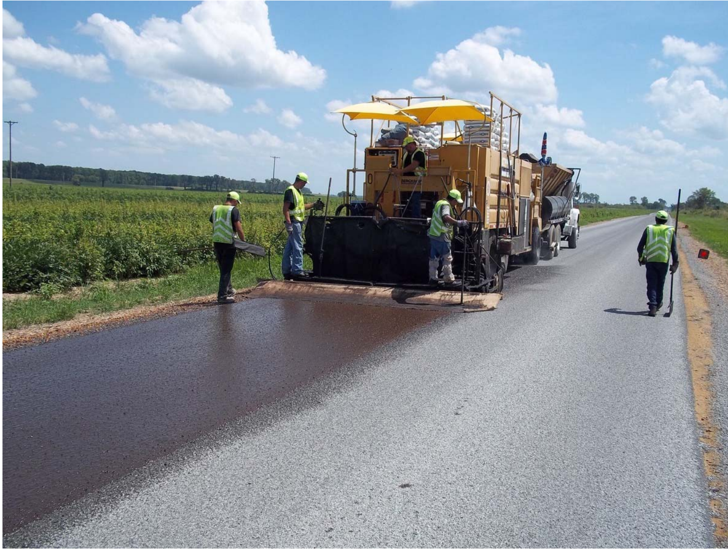
Application of Slurry or Micro Surfacing as top layer
