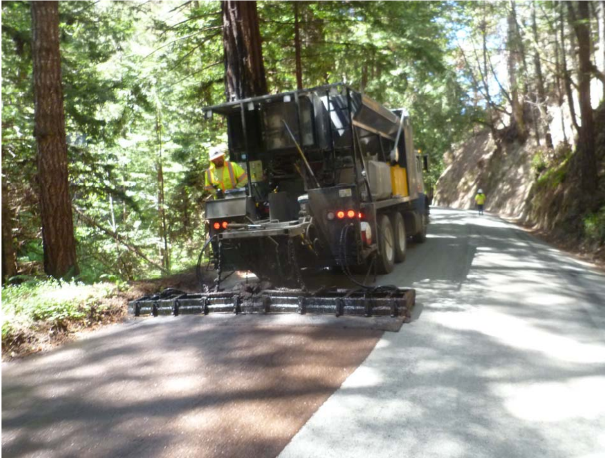
Micro Surfacing application
