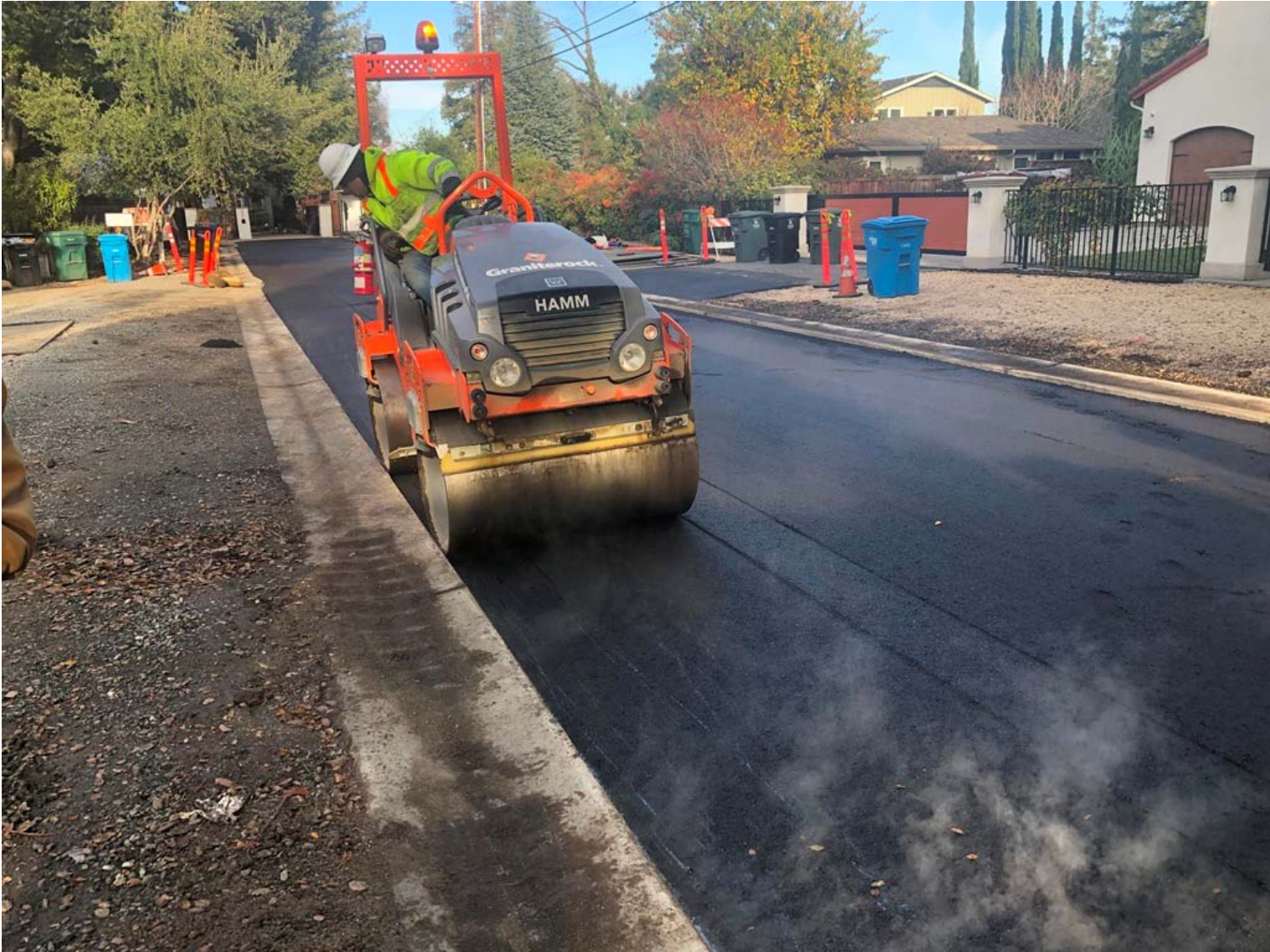
Rolling of new pavement
