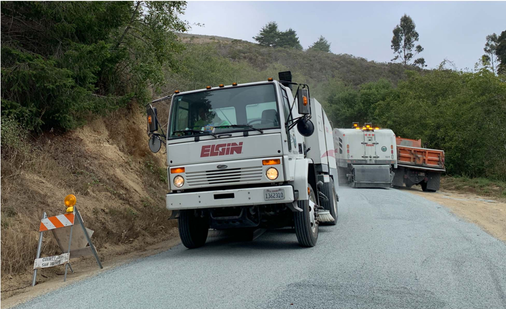
Sweeping of Aggregate
