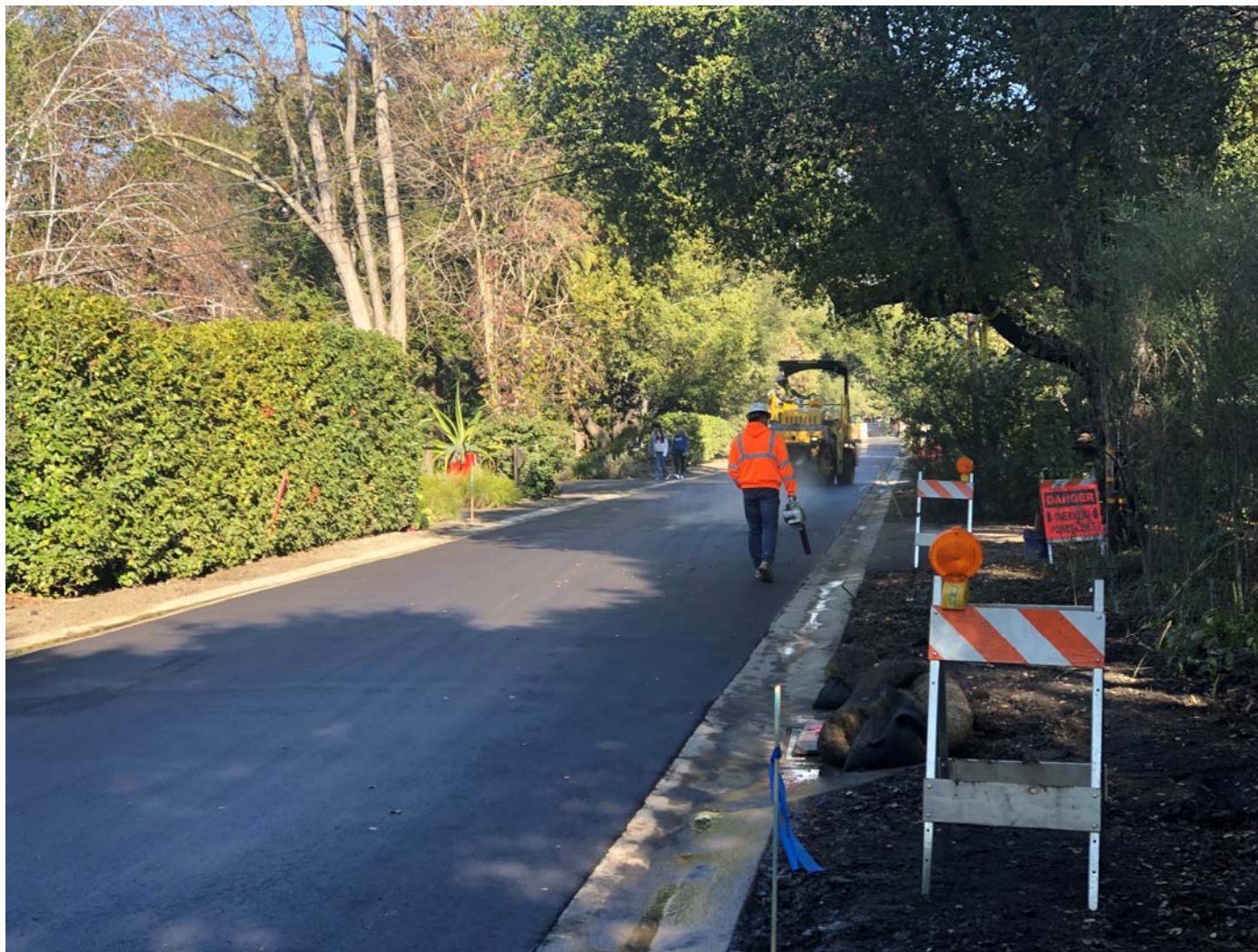
Finished roadway prior to striping
