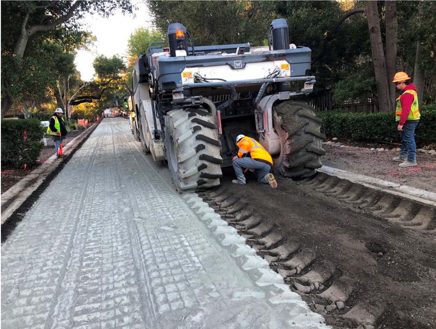
Cement Treatment Machine mixing soil with cement
