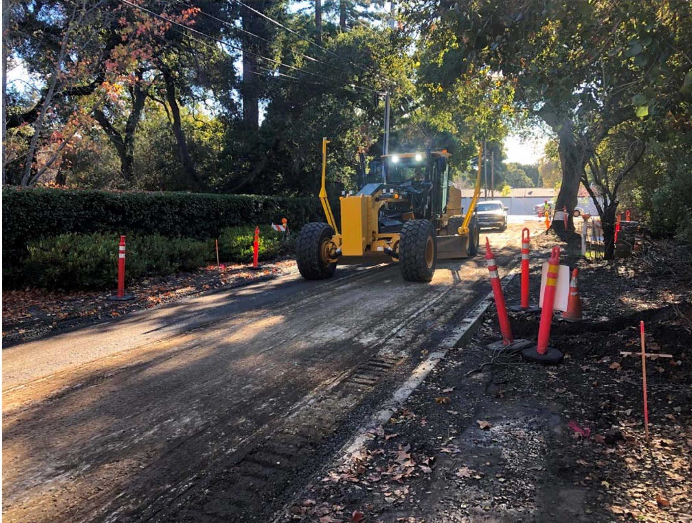
Grading of subbase prior to cement treatment
