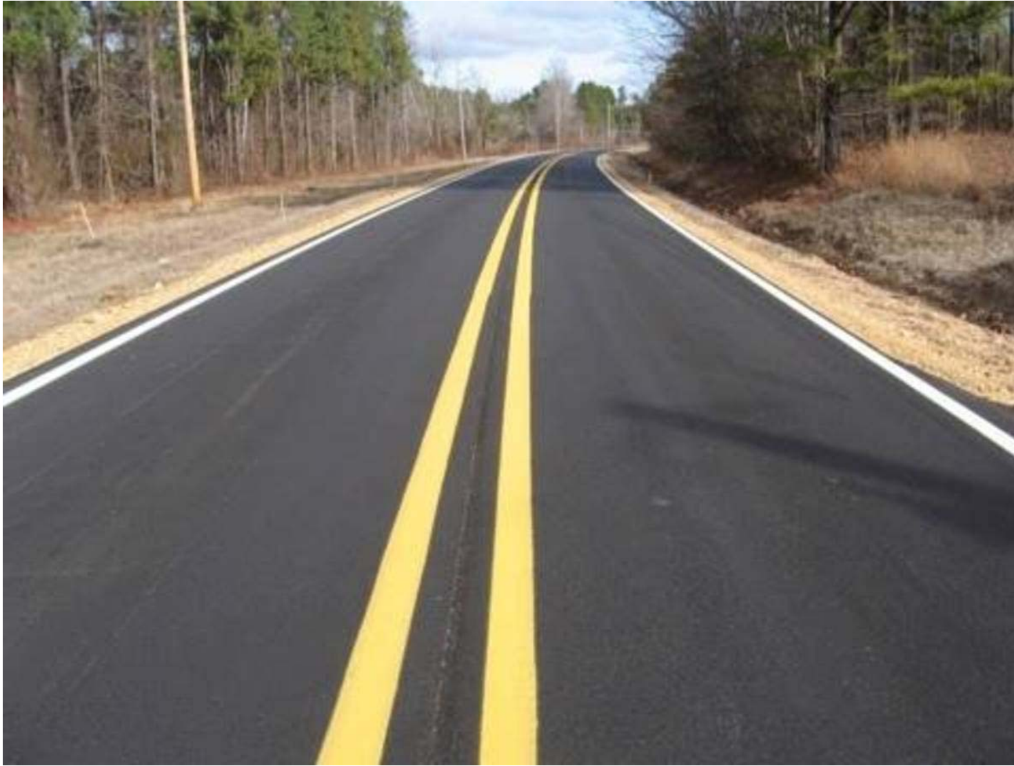
Completed two lane roadway and striping
