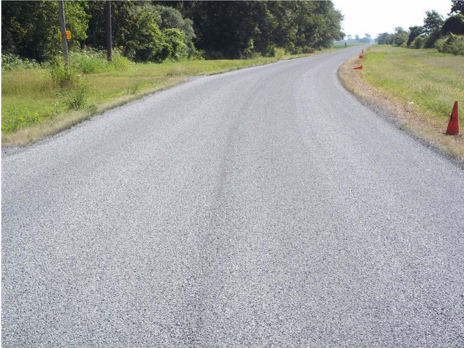
Roadway completed with chip seal application
