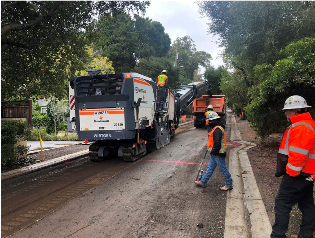
Grinding of existing pavement
