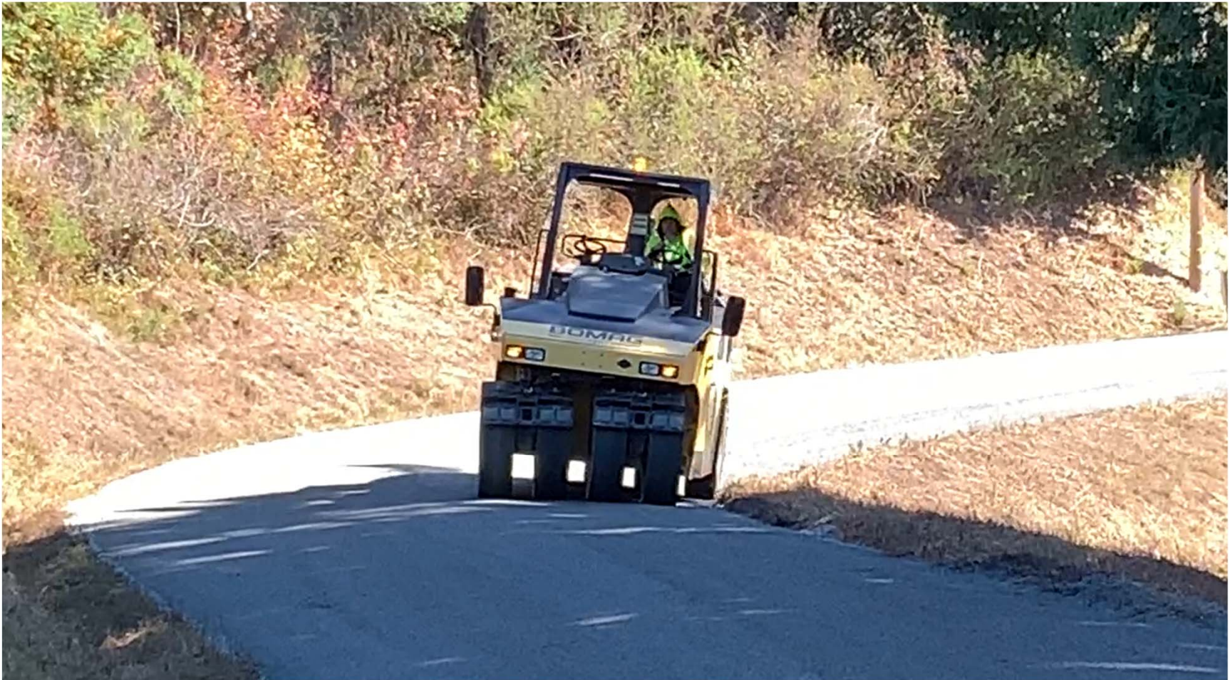
Rolling of Aggregate
