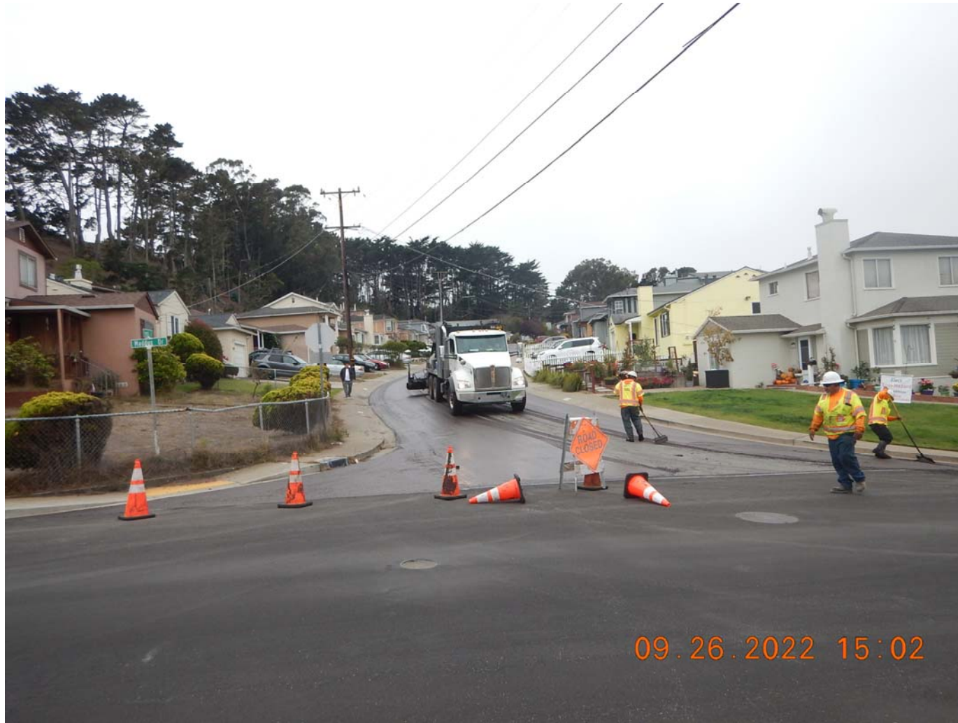
Slurry Application and Hand Work
