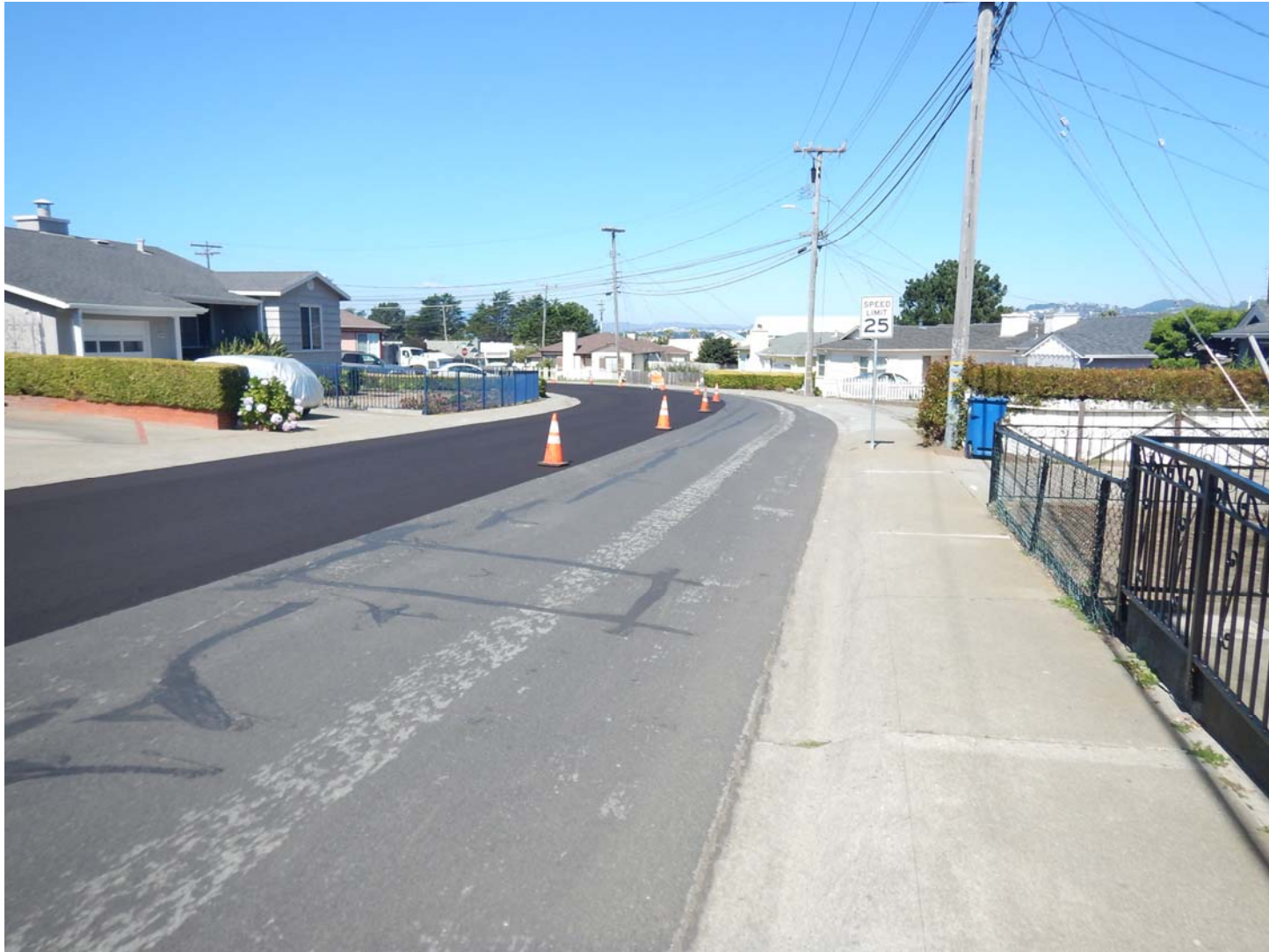
Completed Slurry – One lane to allow traffic
