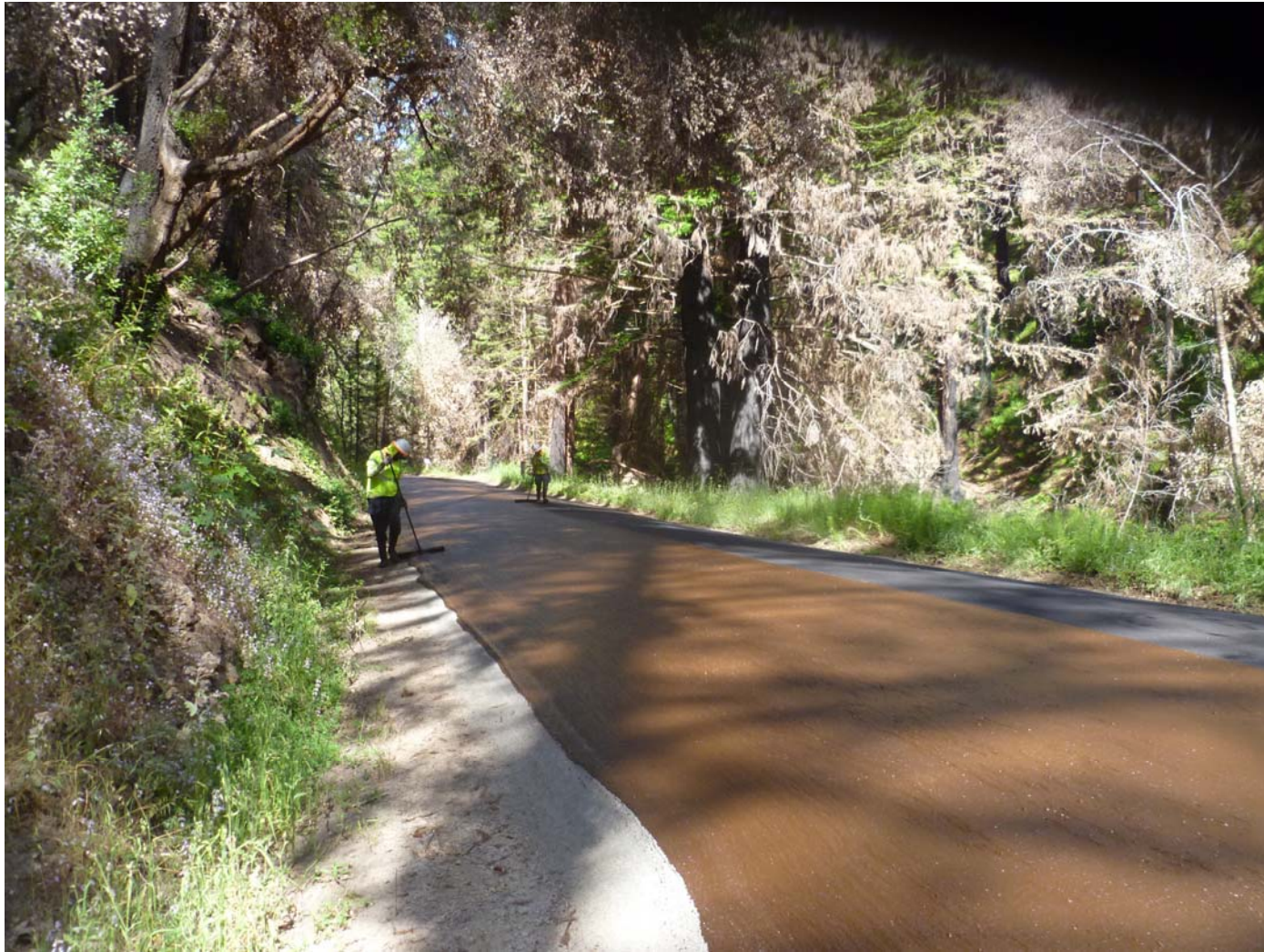
Micro Surface – Hand work on edges of roadway
