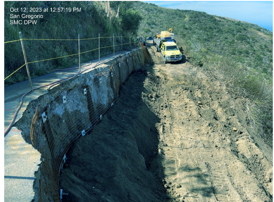
Stage Road – Repair in Progress
