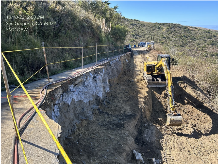
Stage Road – Repair in Progress
