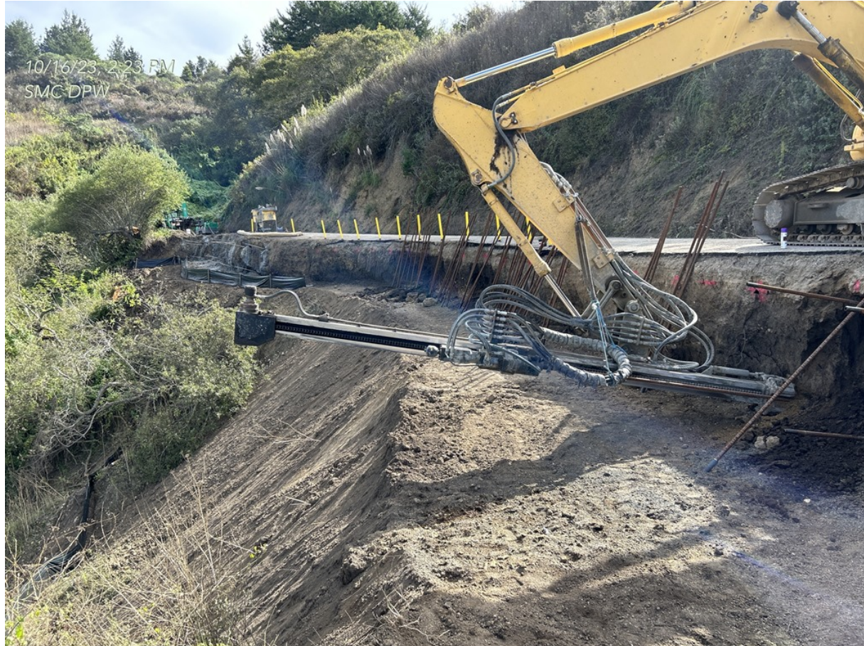
2665 Higgins Canyon Road – Repair in Progress
