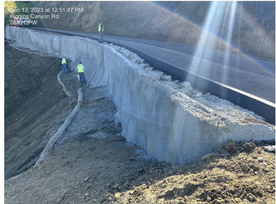
Installation of new soil nail wall
