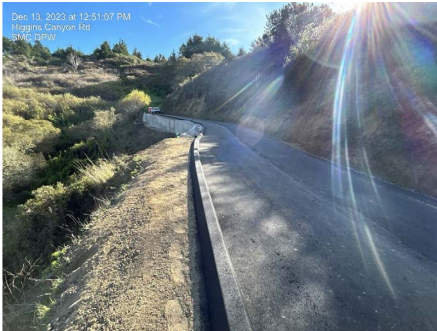
Reconstructed Road with asphalt berm
