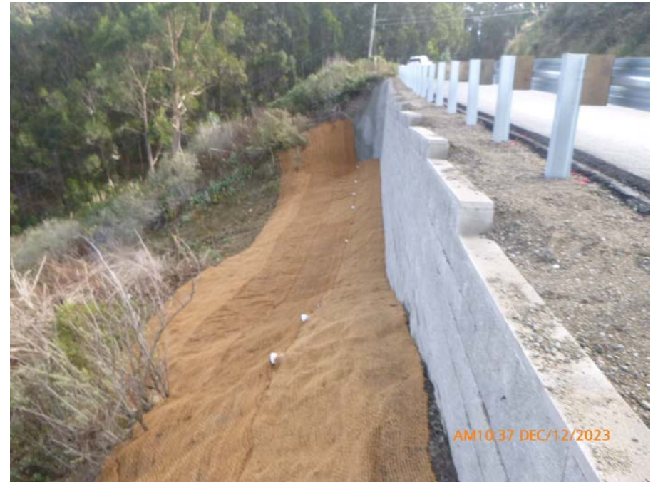
New concrete masonry unit (CMU) wall
