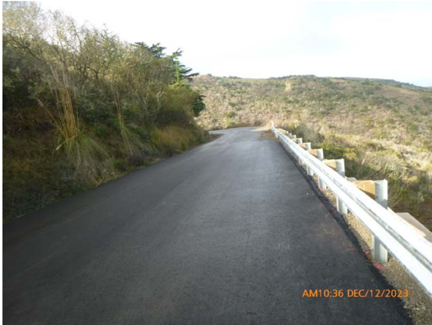
Reconstructed Road with guardrail
