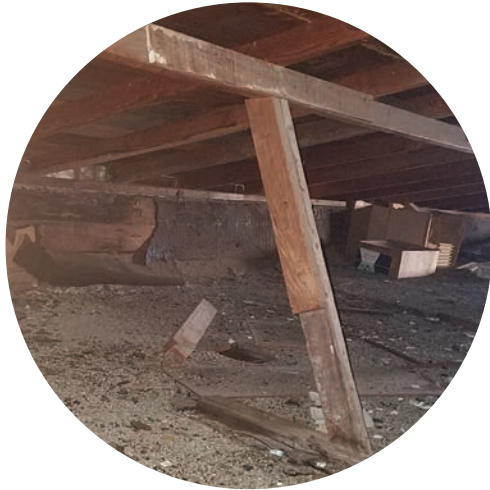
Existing Attic, no insulation
