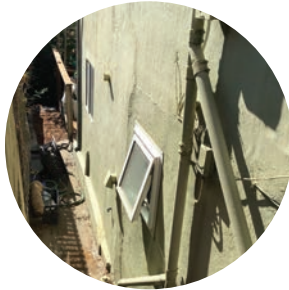
Existing Walls, no insulation
