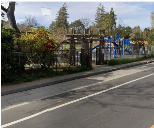
Plate 5 Asphalt concrete (AC) dike
