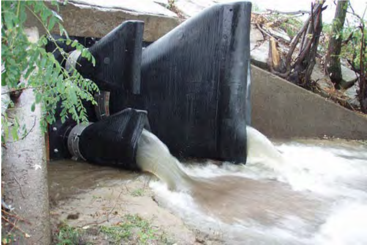
Figure 5-4: Example backflow prevention with duckbill valves.
