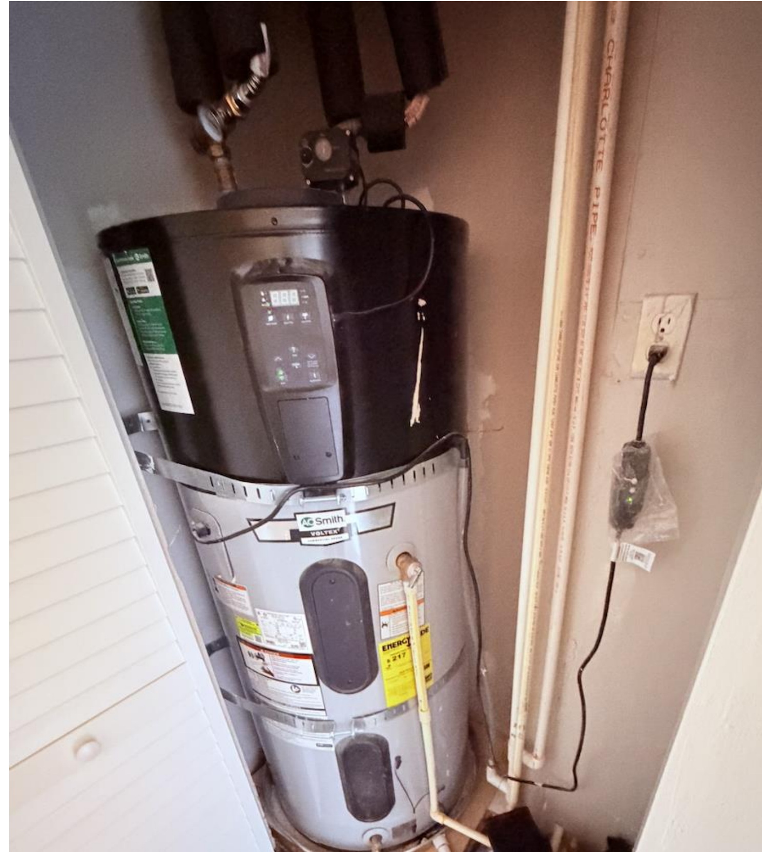
120V Heat Pump Water Heater: High-efficiency unit that plugs into standard outlets.
