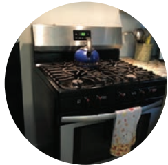
Existing 4-burner 30" propane gas range
