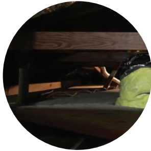
Existing Attic, no insulation
