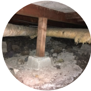
Existing Floor, no insulation
