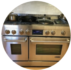
Existing 8-burner 48" gas range
