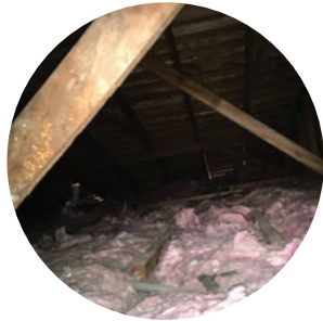
Existing Attic, some insulation
