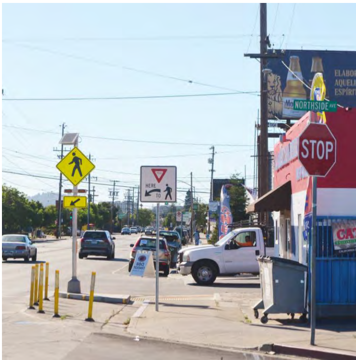
Figure 28: Simulating curb extensions at a crosswalk with safe-hit posts and enhancing the crossing with an RRFB are enhancements that a vision zero program might recommend
