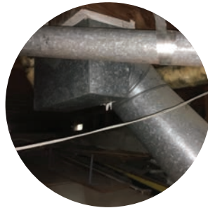
Existing Ductwork, fair condition
