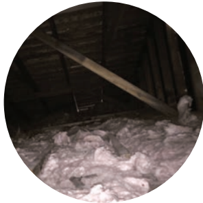
Existing Attic, some insulation
