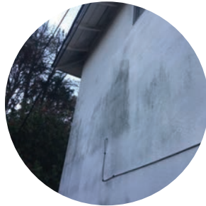
Existing Walls, no insulation
