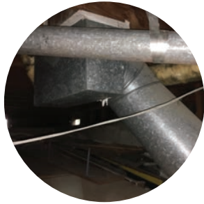
Existing Floor, no insulation
