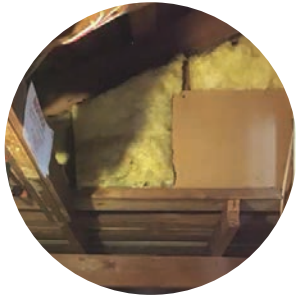
Existing Attic, some insulation
