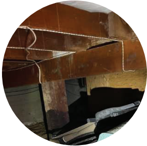
Existing Floor, no insulation
