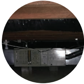
Existing Floor, no insulation
