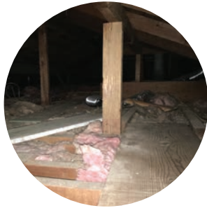
Existing Attic, some insulation
